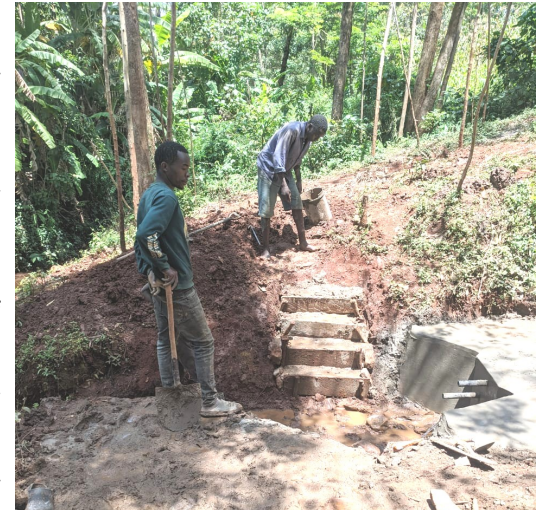
Kabongo spring protection project
